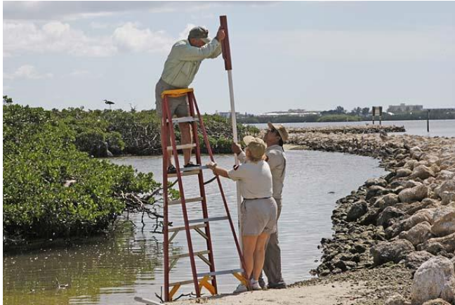
Rick Greenspun uses a pounder to install a post for a “No Trespassing” sign, assisted by Mark Rachal and Ann Paul. Photo: Lou Newman
